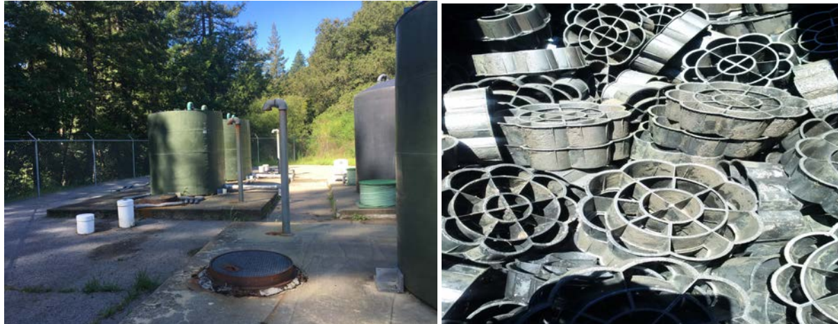
Figure 2: Tank 2 and Trickling Filter Stage One (Left); Random Pack Media Bio-Pac SF 30 (Right)
