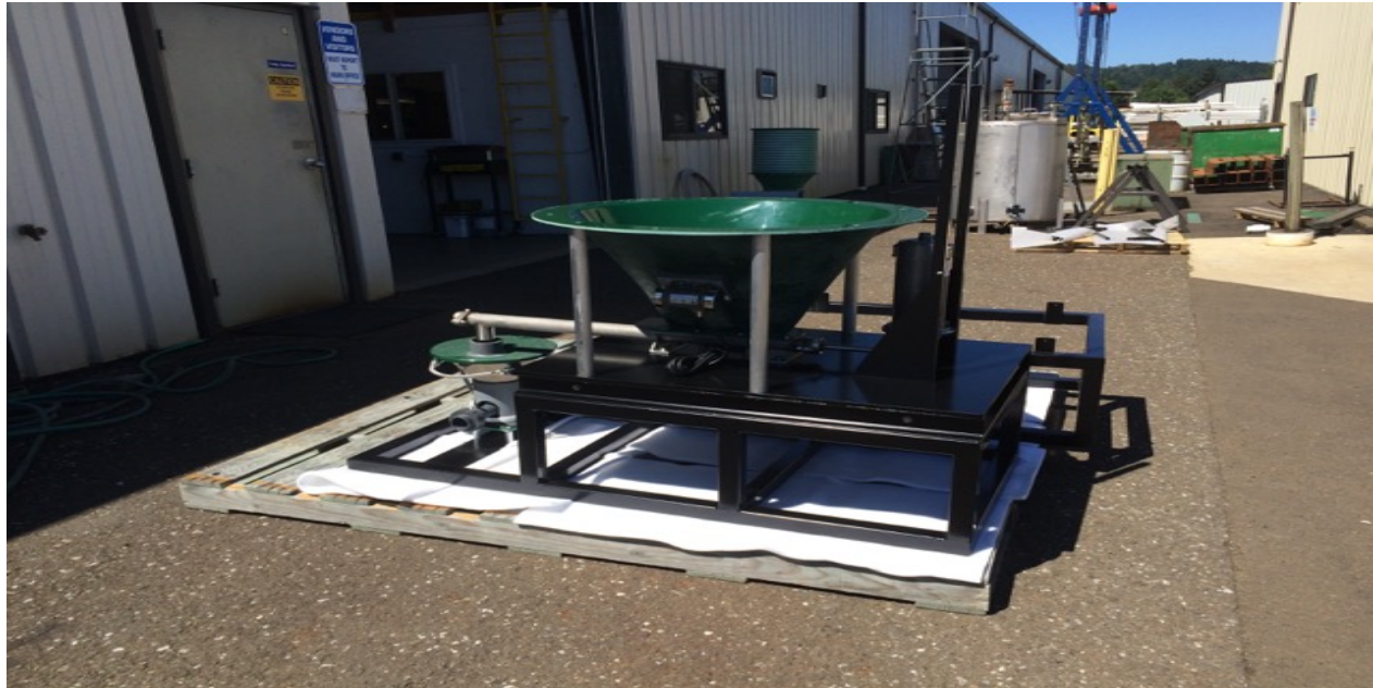
Figure 3: Alkalinity Feed System (typical)
